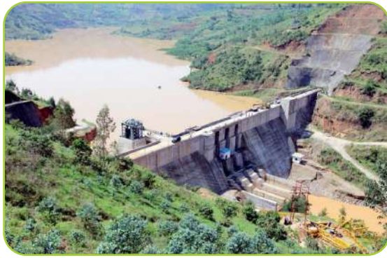
Fig 10.4 Dam on Nyabarongo River.
